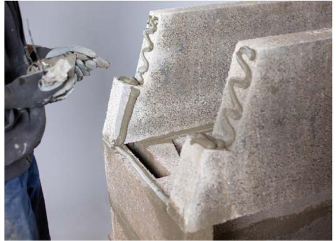
Apply lip glue to the joints on the sides of the front and rear panels of the gather.
