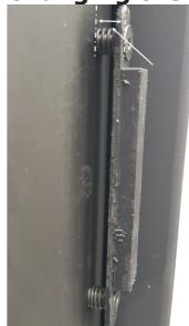
To change the pull in the door, adjust the two magnet modules.
